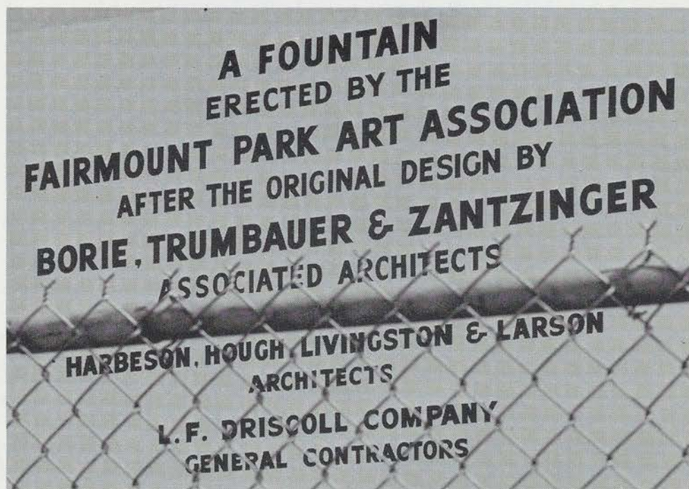
Sign erected during construction of Eli Kirk Price Fountain
