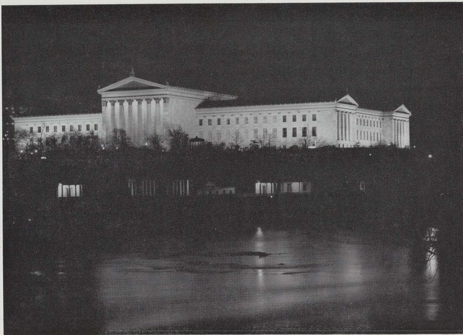
Photograph by C. V. D. Hubbard Floodlighting of west and south facades of Philadelphia Museum of Art. Installed by the Fairmount Park Art Association.
