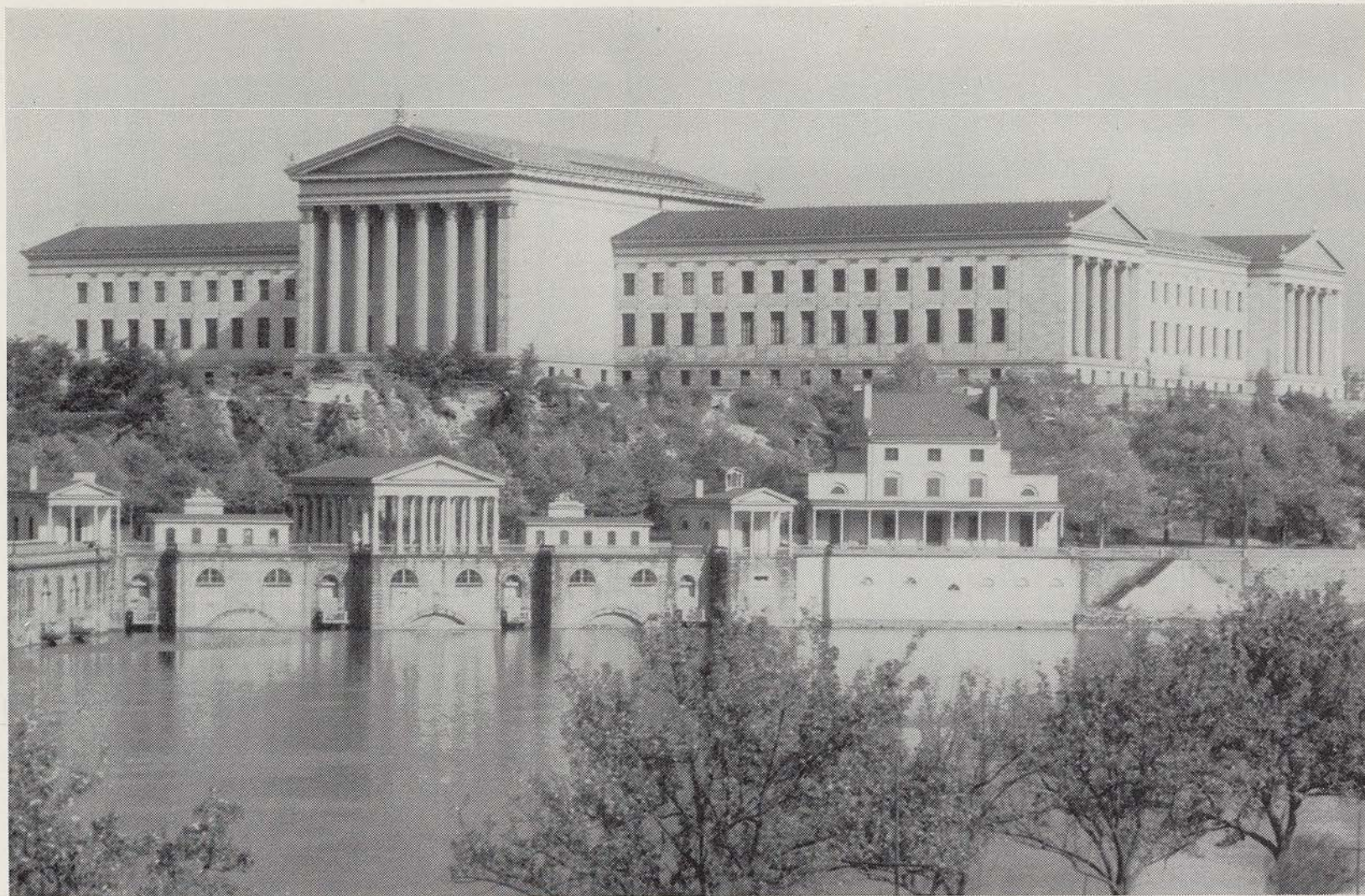
The water works designed by Frederick Grauff in 1812. Above the Philadelphia Museum of Art.
