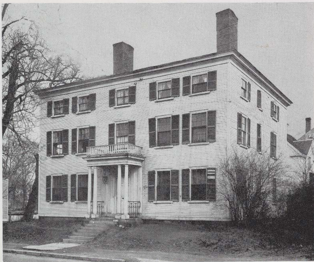
Captain Barnes House, built in 1807. Portsmouth, N. H.
