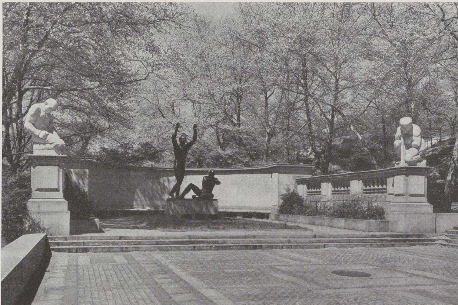
NORTH EXEDRA OF ELLEN PHILLIPS SAMUEL MEMORIAL FIRST COMPLETED UNIT ON THE EAST RIVER DRIVE
