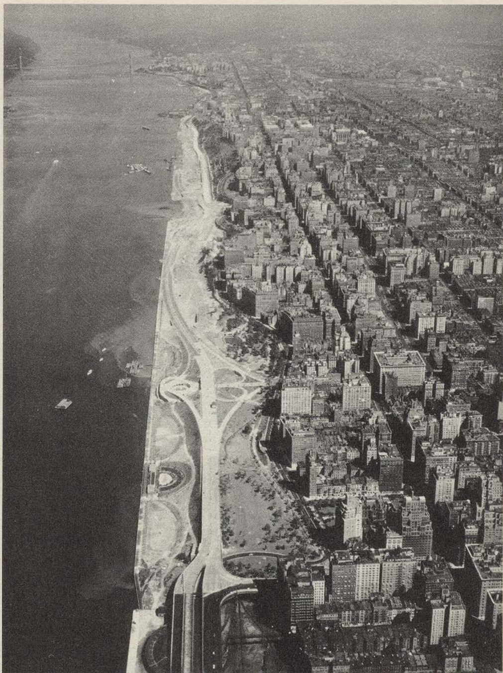
HENRY HUDSON PARKWAY—AIR VIEW OF WEST SIDE IMPROVEMENT FROM 72ND ST. TO GEORGE WASHINGTON BRIDGE
