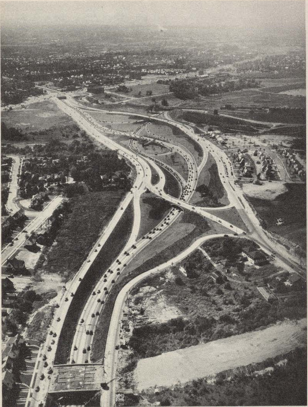
SHOWING INTERSECTION OF GRAND CENTRAL PARKWAY INTERBORO PARKWAY AND GRAND CENTRAL EXTENSION
