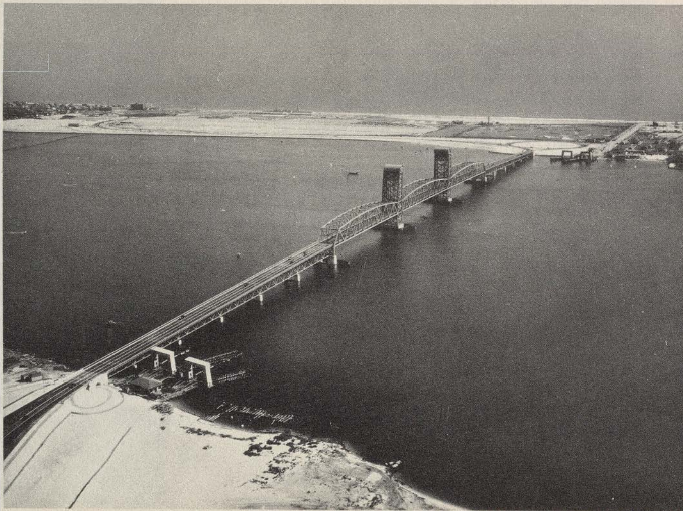
PARK DEPT. NO. 12536, MARINE PARKWAY BRIDGE LOOKING TOWARD JACOB RIIS PARK
