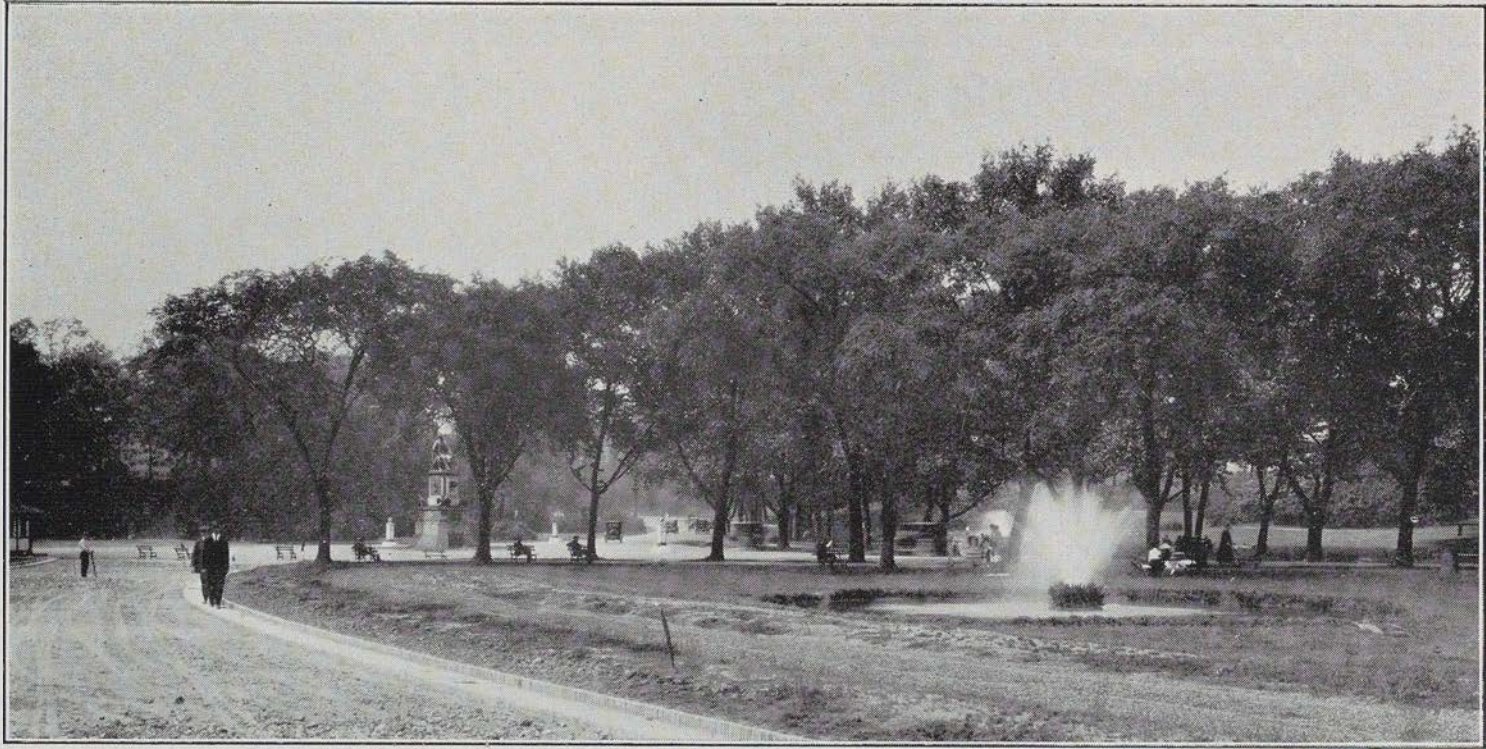
ONE OF THE TWO FOUNTAINS SHOWN IN THE PREVIOUS ILLUSTRATIONS STILL IN ITS ORIGINAL LOCATION. Note the development of the Park.
