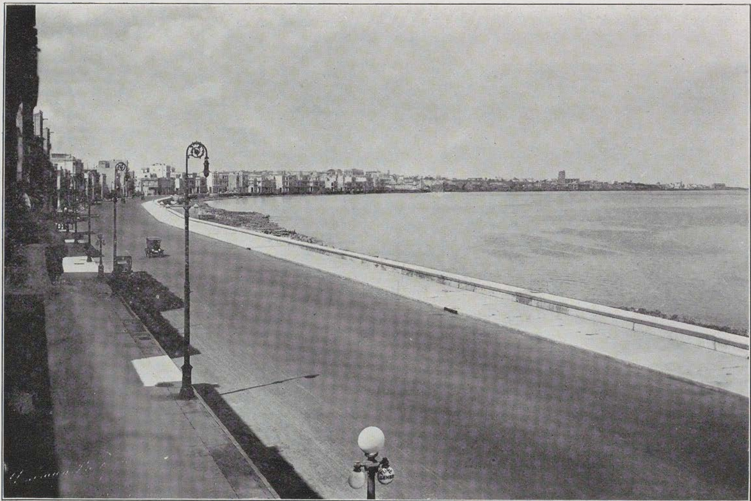
THE MALECON, HAVANA, AFTER IMPROVEMENT. Philadelphia should likewise reclaim its Schuylkill Water-front.
