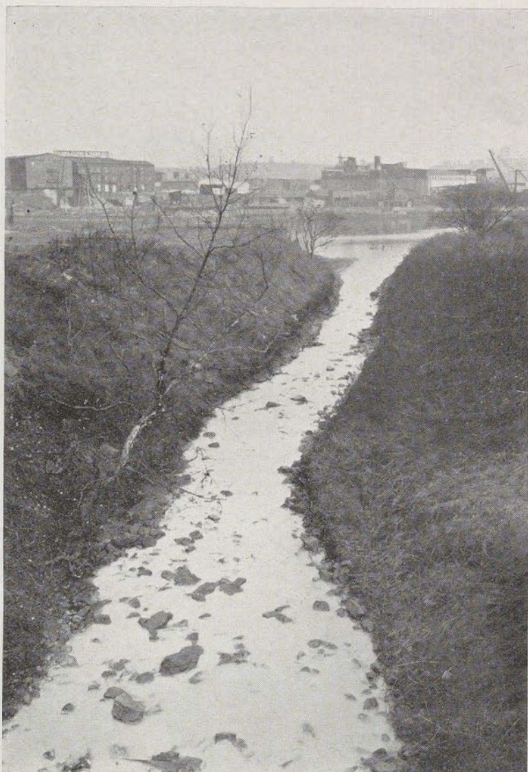
VIEW OF AN OPEN SEWER, WEST BANK OF THE SCHUYLKILL, JANUARY, 1921
