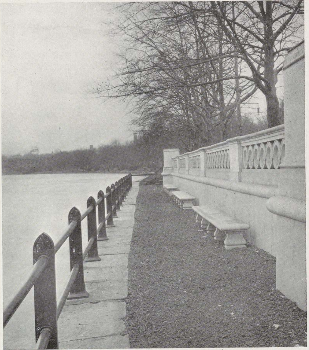
FULL-SIZE STAFF MODEL OF THE BALUSTRADE OF THE PROPOSED ELLEN PHILLIPS SAMUEL MEMORIAL, AS ERECTED BY THIS ASSOCIATION ON THE EAST RIVER DRIVE BELOW GIRARD AVENUE BRIDGE, IN FAIRMOUNT PARK. VIEW FROM THE RIVER-WALL.
